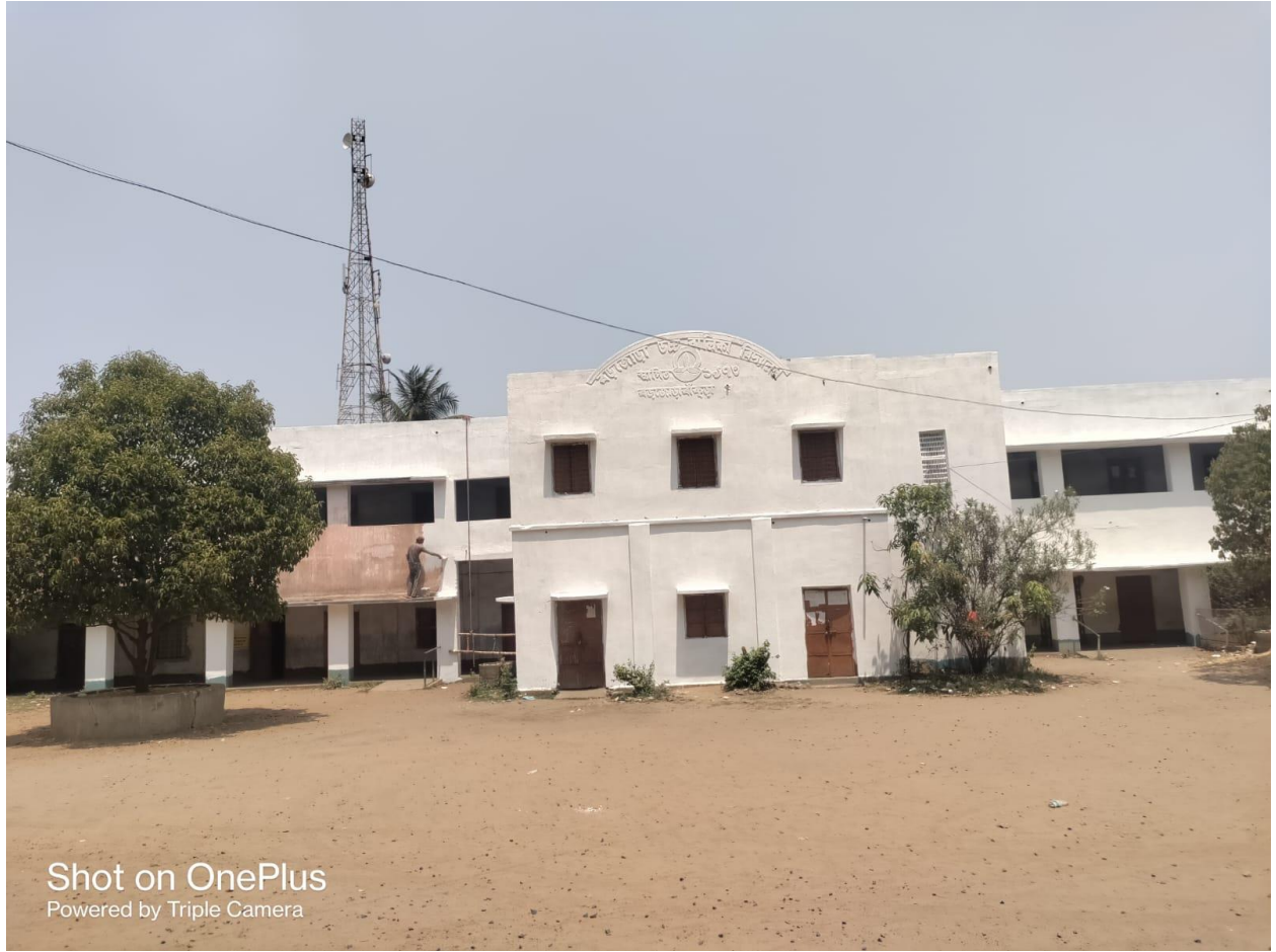
Painting work at School Building
